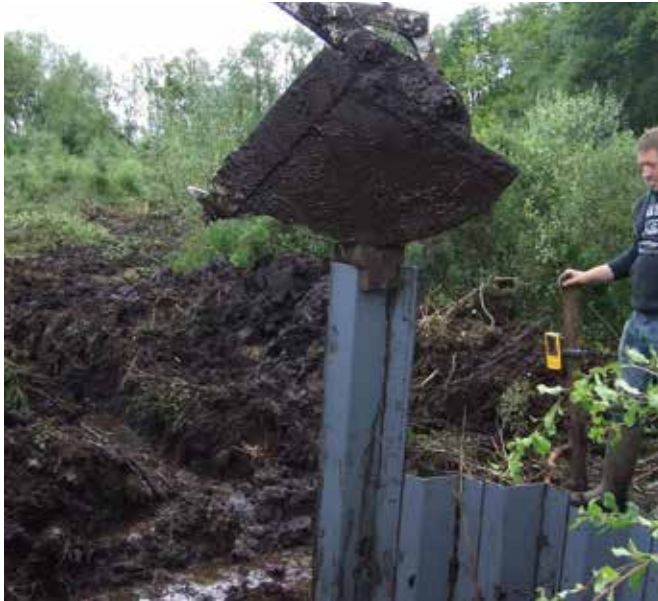
Piling being installed at Wem Moss NNR. Photography by Matt Jones.
