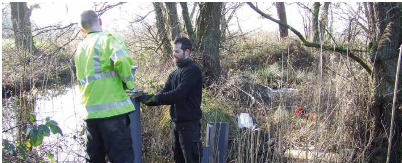
Farm Advice Case Study - artificial water management on the Cholmondeley Estate using plastic piling. Photography by Matt Jones.
